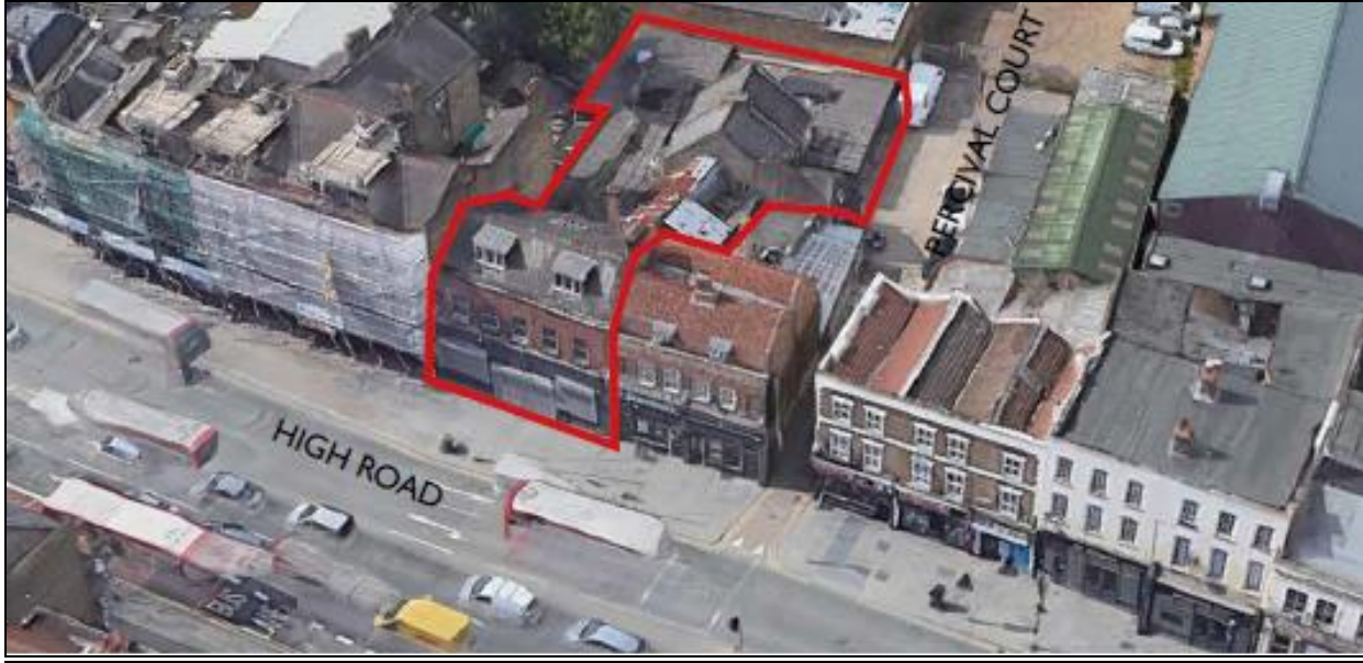
The site - No. 807 High Road
