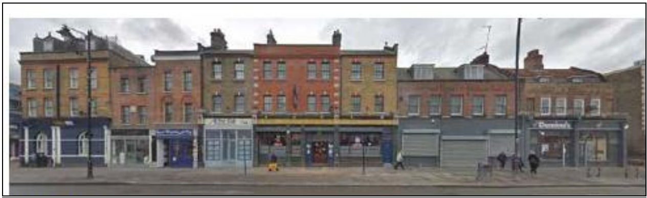
Existing High Road elevation
